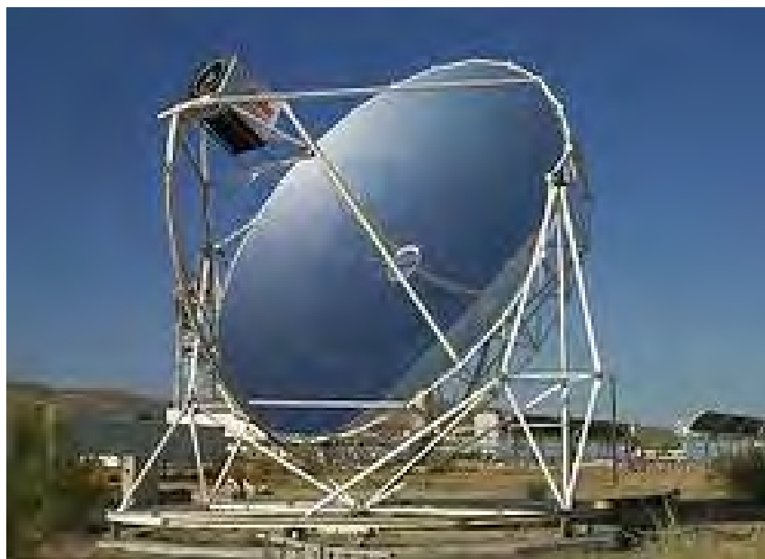
Fig. 5. Dish-Stirling system for electrical energy produced.
