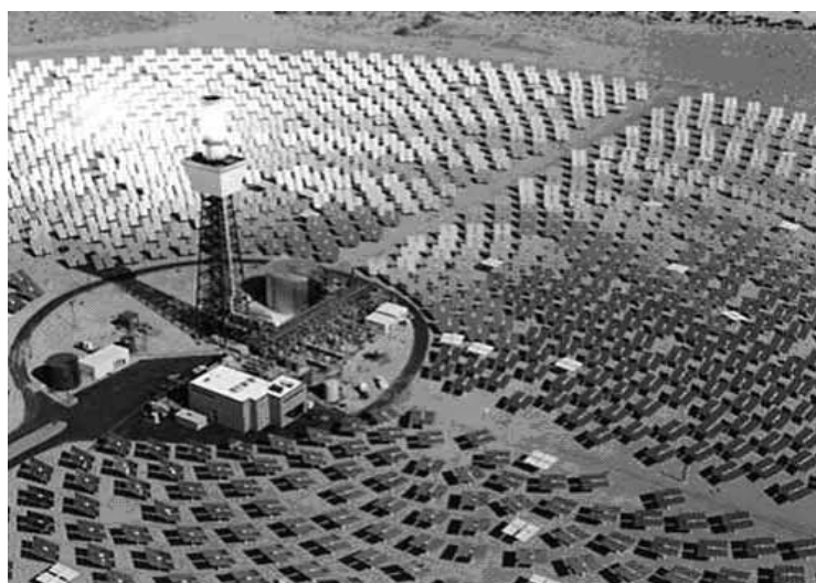
Fig.2. Electrical energy generation with solar tower system
